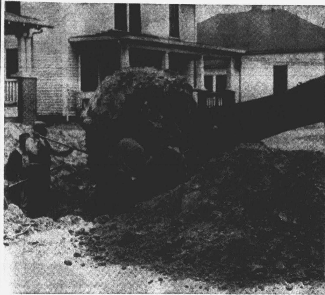
A city crew spent several days last week "uprooting" trees on Cotanche Street between Second and Third Streets. The old trees were on city property, along the curbs of the street, and were cleared away because the roots interfered with the pavement. (Reflector Photo by Robert C. Smith).
