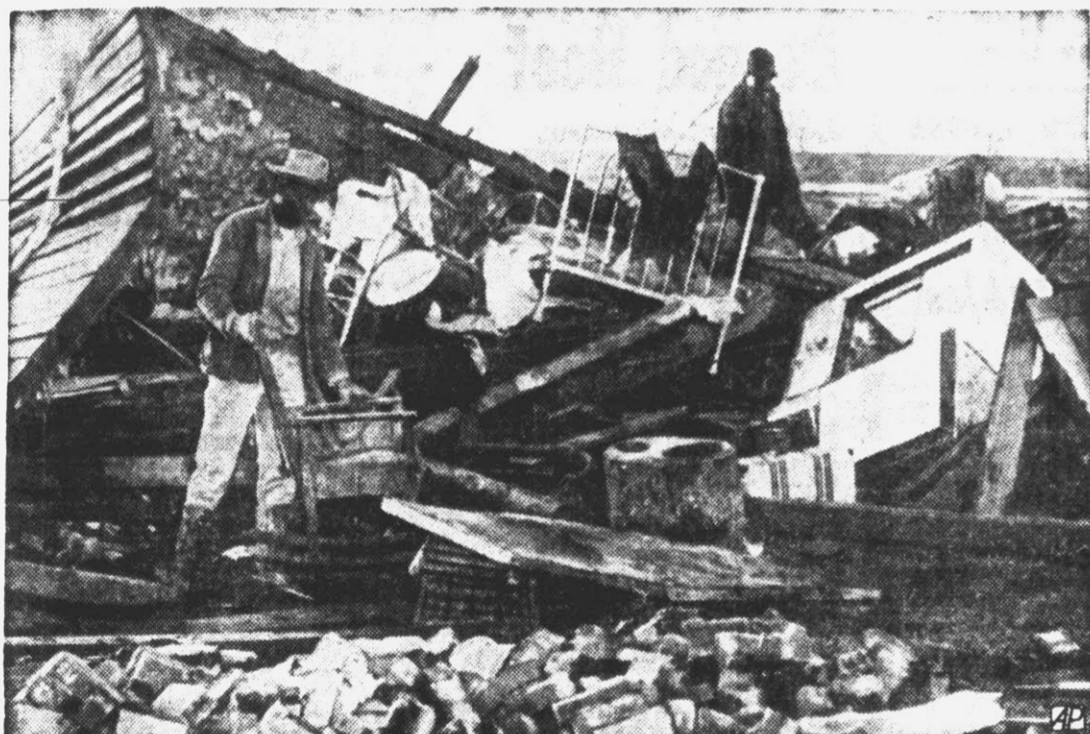
IN PATH OF DESTRUCTION: — Henry Hill, at right, searches through the wreckage of his home in Commerce Landing, Miss., after a tornado struck, killing his father, Cleveland, 58, and a nephew, Albert Hill, 21. The giant corkscrew winds that ripped through Mississippi, Arkansas and Alabama left 31 dead—28 of them in Commerce Landing—and about 100 injured. Man at left is unidentified. (AP Wirephoto).
