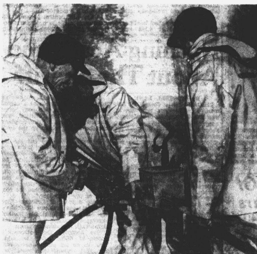
Preparing for fresh fall, Stanley Galewaler holds aluminum laterals as Monvo Bosch and John Eck plug water and air lines into box head.
