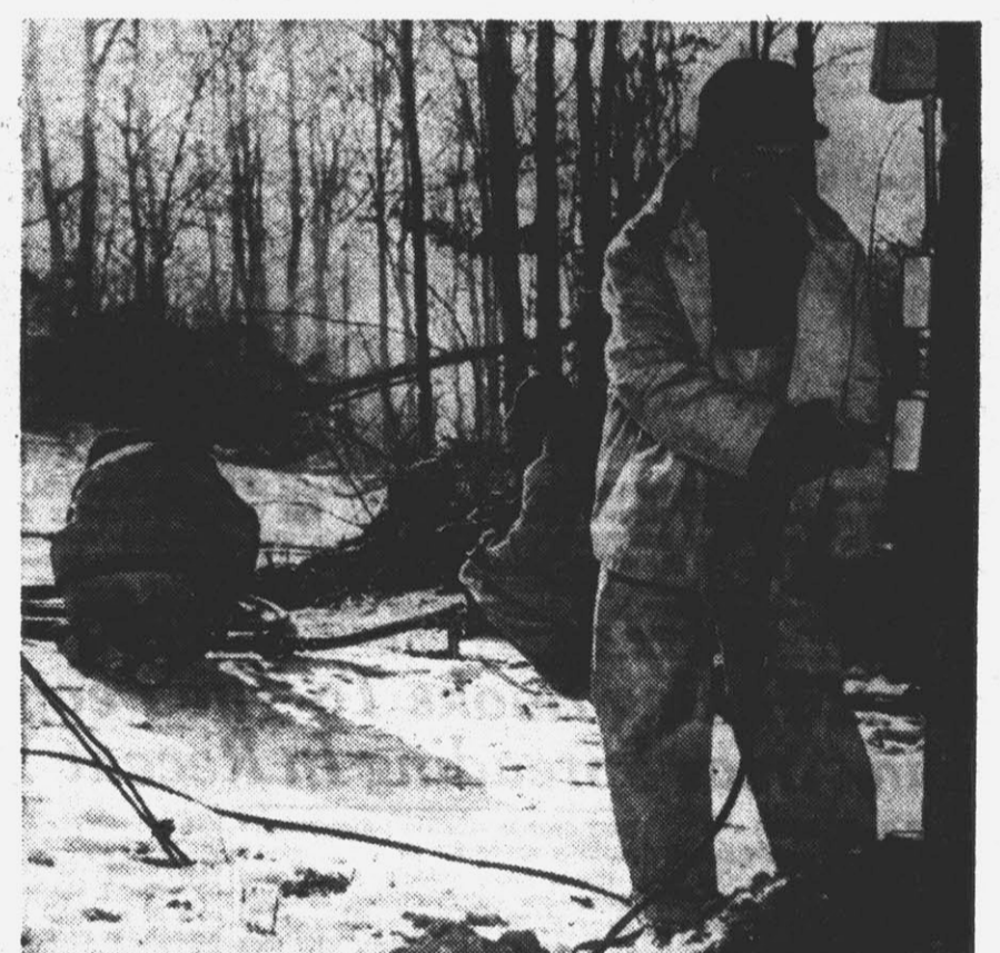
Lateral box heads are heated to prevent water from freezing in nozzles. Monvo Bosch puts "heat" on by plugging in electric line.
