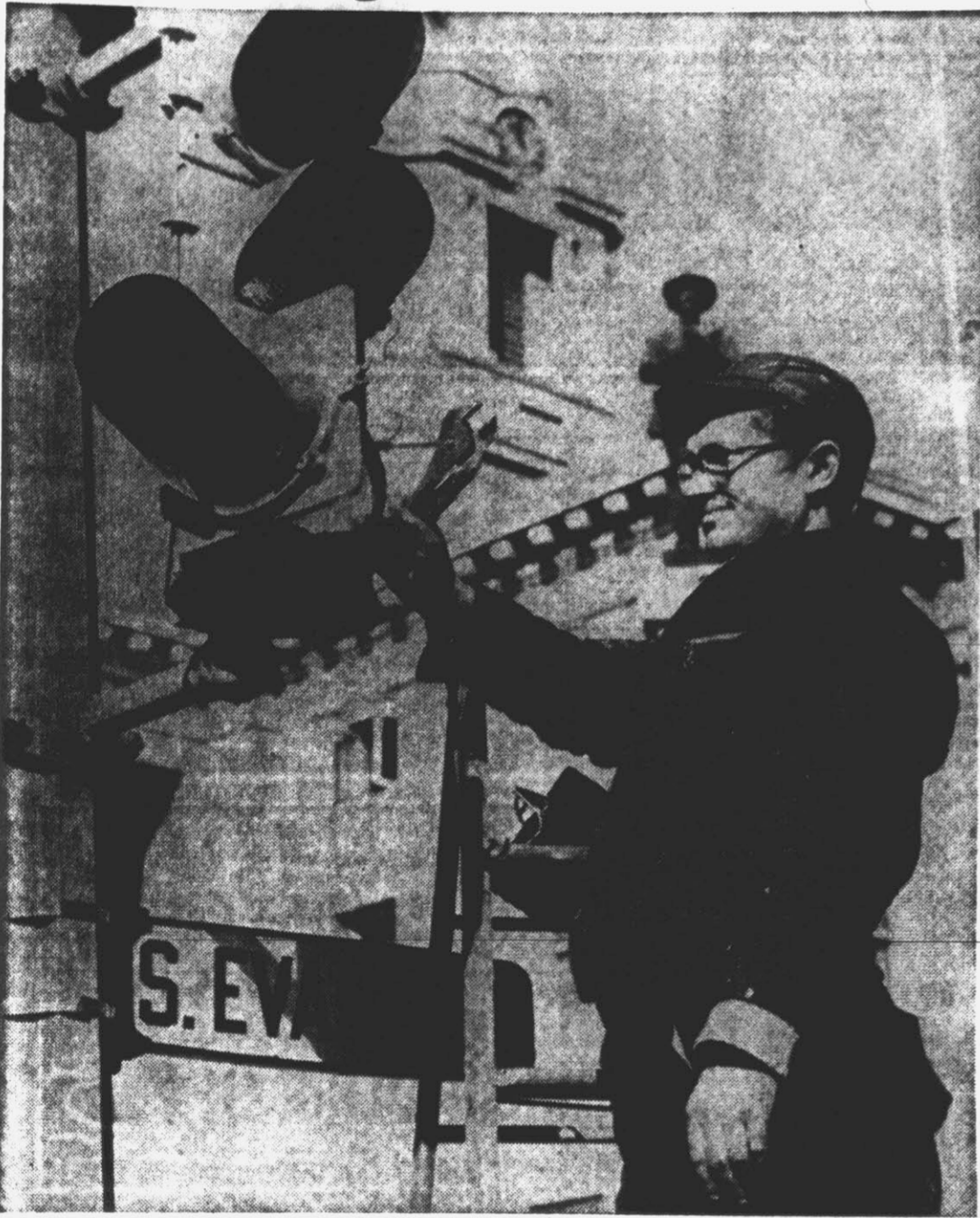
A street department workman is shown above as he changes a green lens in one of the downtown traffic signals. Arrows on the new lens indicate the proper directions in which motorists may turn on the one-way streets. Where green lenses remain turn may be made in any direction.
