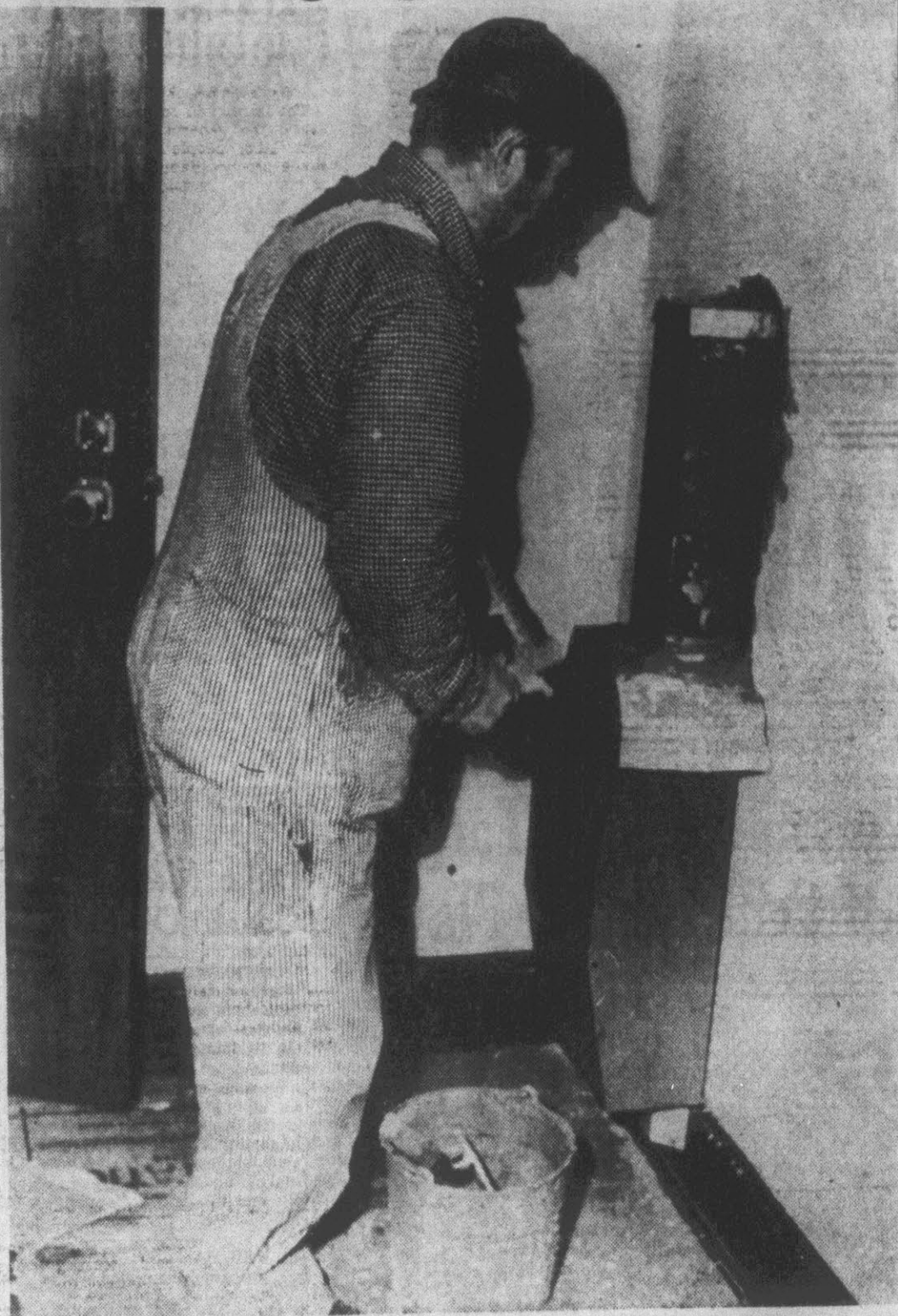
A workman is shown above as he plasters the new depository into place at city hall. The rear view above shows the vault portion of the device. The deposit slot is in the east hallway at the municipal building. Greenville Utilities customers will be able to pay their bills at any time day or night since the hall will be kept open for their use. (Reflector Photo by Alvin Taylor).
