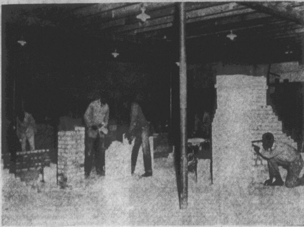
Featured in the curriculum at C. M. Eppes High School is a class in bricklaying. Here some of the students are shown at work. There are 22 enrolled in the class with Herman R. Foust as instructor. (Reflector Photo by Edwina Haymes).
