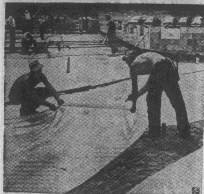
PLASTIC FILM is stretched over a sand bed to prevent punctures. Reinforcing steel is laid on top. Concrete poured over this is permanently sealed against moisture.
