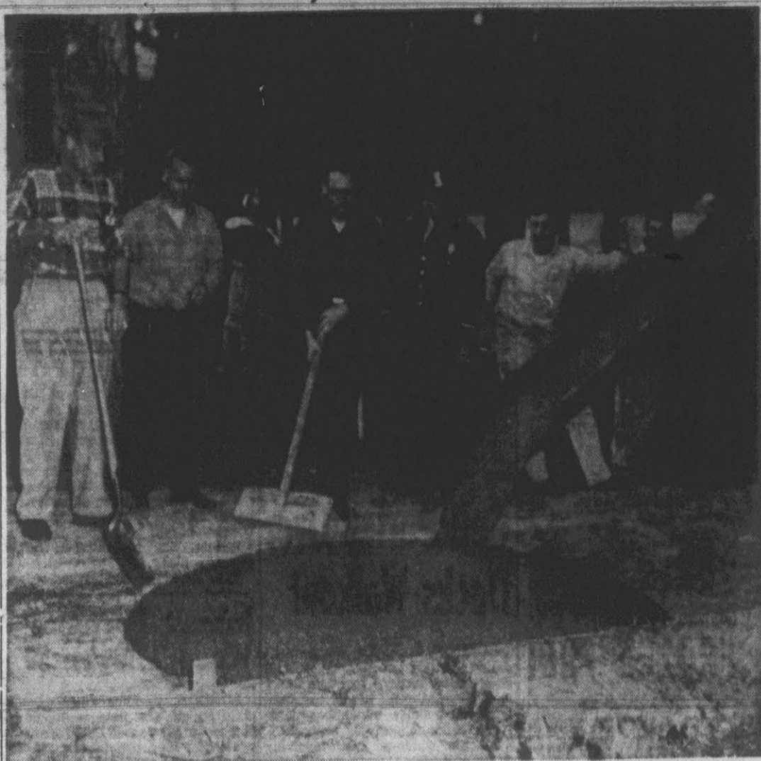
Members of the local Red Men's tribe look on as concrete is poured into the form at Elm Street Park for a 16 foot barbecue pit. The pit is to be used for a Western style barbecue to be sponsored by the Red Men on November 12 and will be left at the park. (Reflector Photo by Alvin Taylor)
