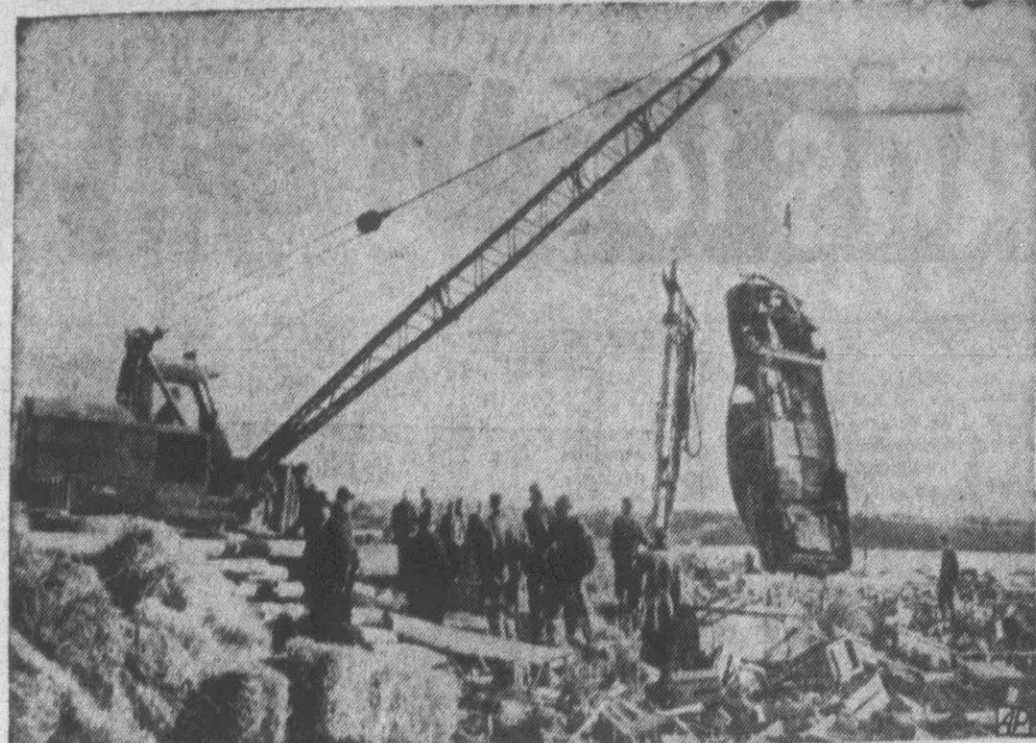
"OPERATION CLEANUP"—Now that the water has receded, crews of men and machines have started the grim task of cleaning up the destruction left in the wake of "Hurricane Hazel" in and around Toronto, Canada. Here a crane pulls a car loose from what once was fertile farm land. Water covered more than 7,000 acres around Toronto, making 3,000 persons homeless. Damage was estimated at $10,000,000. (AP Wirephoto).
