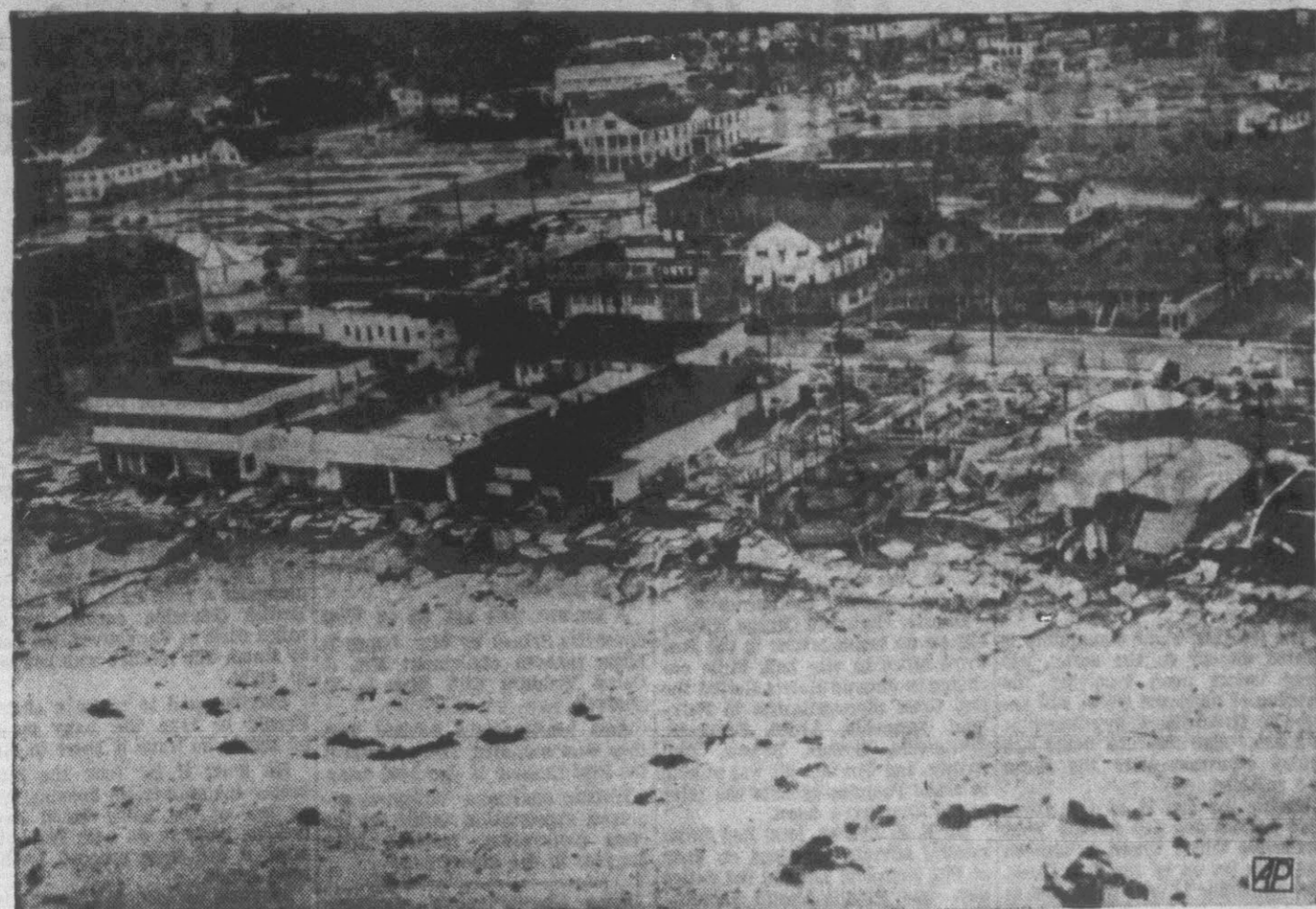
FLATTENED BY HURRICANE HAZEL:—An amusement park at Myrtle Beach, S.C., lies in ruins after hurricane Hazel hit the coastal resort. Pavilion at far left was badly damaged along with most of the beachfront buildings. Photo was made by Charlotte Observer photographer Virgil Patterson who flew over the area. (AP Wirephoto).
