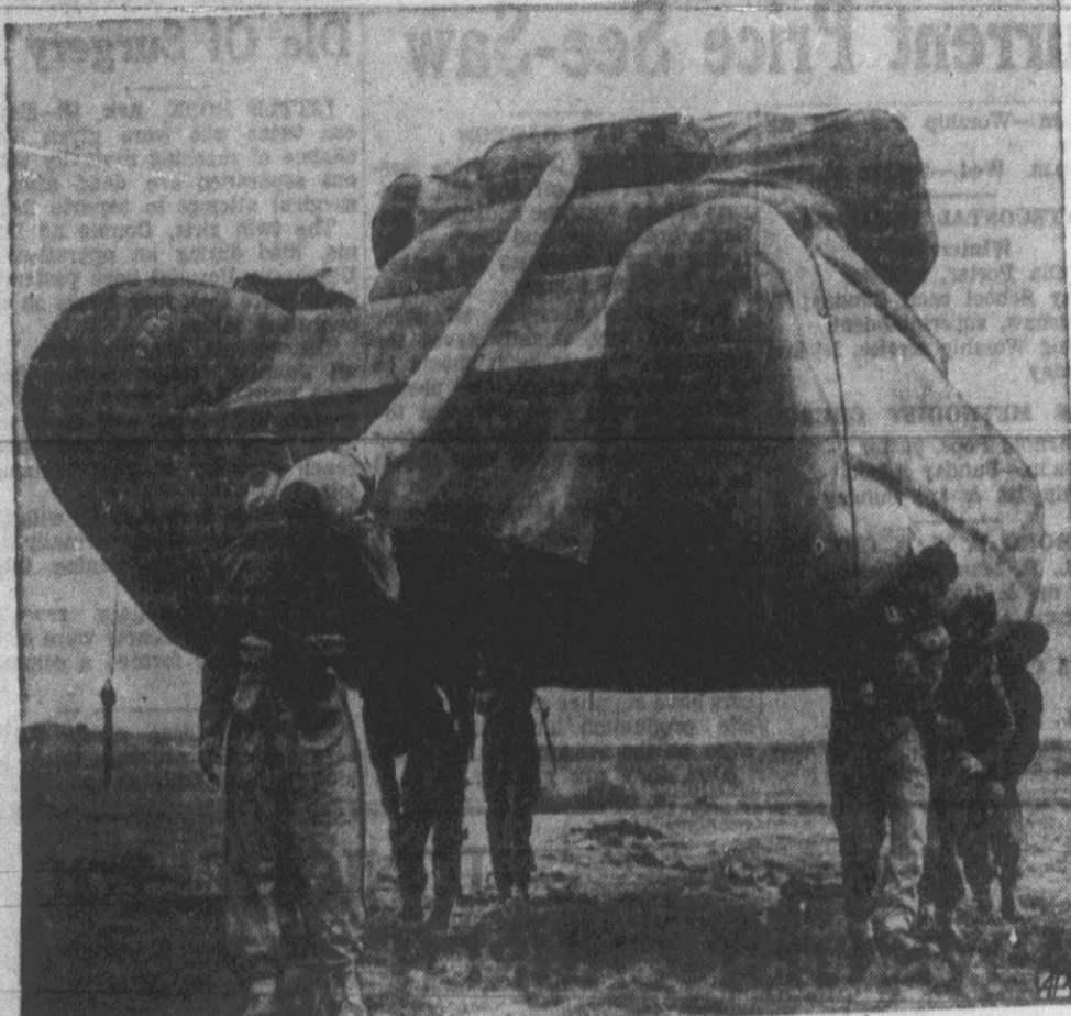
PORTABLE TANK — British Home Guardsmen put their shoulders to inflated dummy tank, simulated weapon designed to confuse enemy, in exercises at England's Salisbury Plain.
