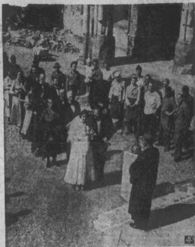
WORK STOPS FOR WEDDING —Workmen repairing Kaiser Wilhelm Memorial Church in West Berlin watch wedding in rubble, first held since church was bombed in 1943.
