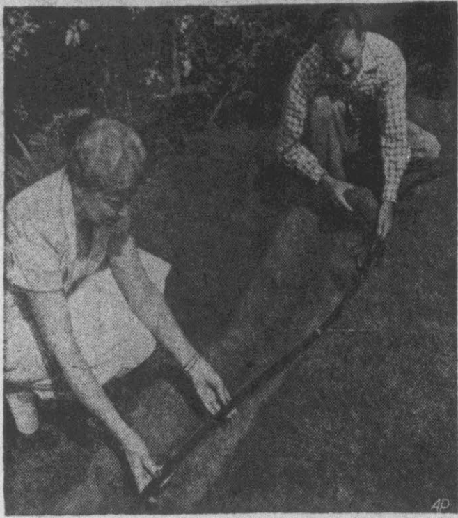
FLEXIBLE PLASTIC pipe, with sprinkler heads spaced for even coverage, is easy to lay under sod.
