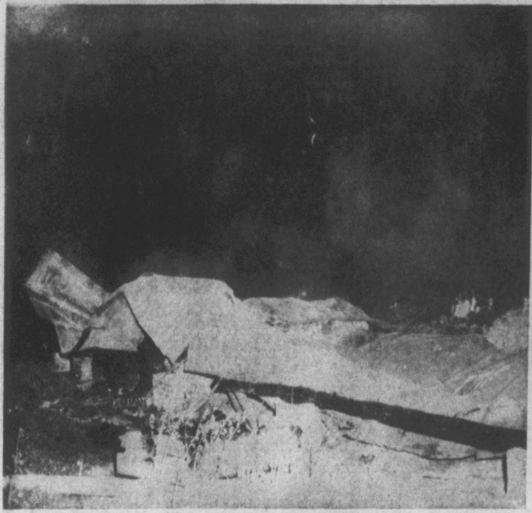
Pictured above is a portion of the smoldering ruins of a tobacco pack house located on the Smallwood farm on the Falkland Highway. Five families had varying amounts of tobacco stored in the 56 by 40 foot barn. Loss of the tobacco alone was conservatively estimated by Atlas Wooten, overseer of the farm, at $10,000. K. R. Wooten of Falkland owns the farm. (Reflector Photo by Alvin Taylor)
