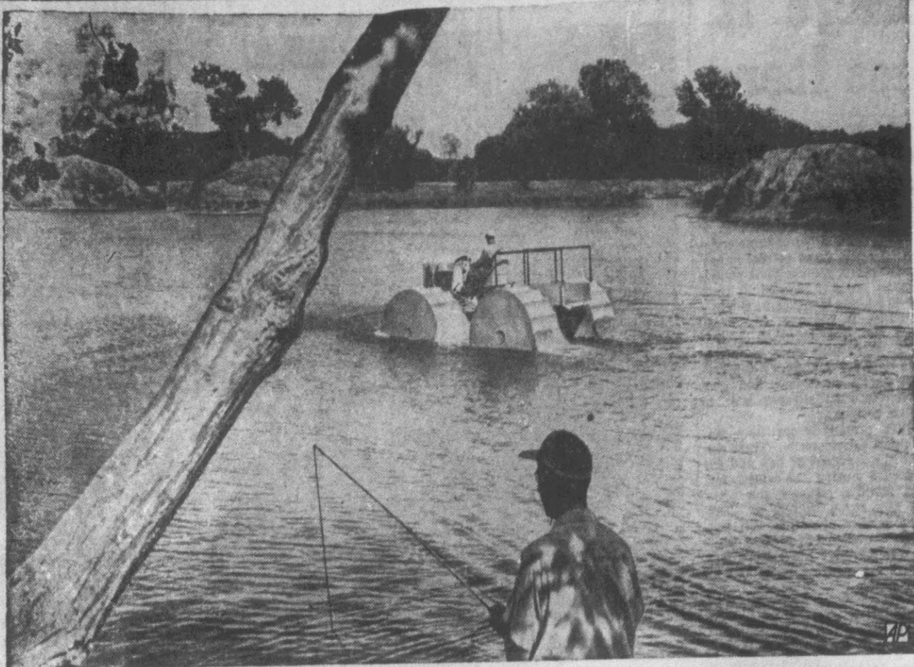
WATER WAGON —A "swamp buggy," designed and built in Kansas for use in Minnesota pipeline construction projects, gets a deep-water test in Cave Lake, near Dodge City. It can run on hard or soft ground, in or out of water.
