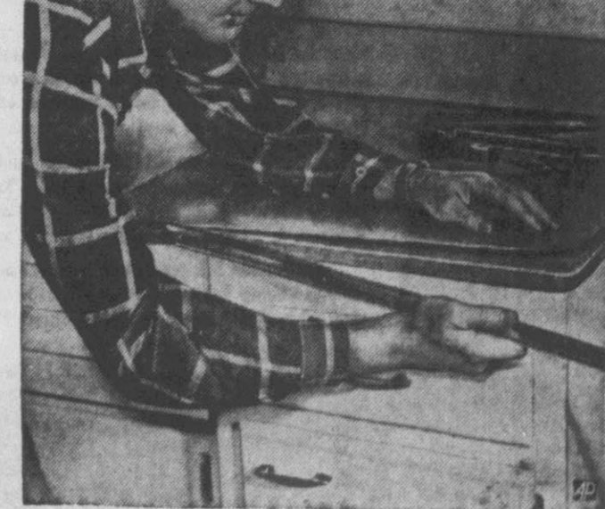
NEW THIN plastic covering for countertops is curved to make it lie flat under tension from metal trim.
