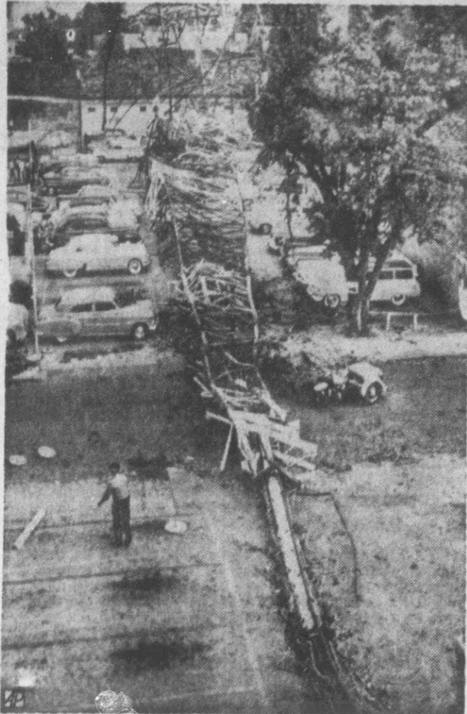
TWISTER PULLS TV TOWER —A twister during a sudden windstorm swooped down on the 435-foot tower behind the WALA-TV building in downtown Mobile, Ala. and sent the tower sprawling to the ground. Miraculously it fell between two rows of cars in a parking lot—the only way it could have fallen without crashing into a building. Several cars were damaged but no one was hurt. The 85-foot television antenna on top of the 350-foot tower proper weighs 4½ tons. The tornado also tore roofs off several buildings and blew out windows in many buildings. (AP Photo)
