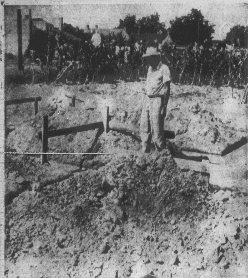
Graven Hughes looks over the foundation for the new $60,000 building now being constructed by the local Moose Club at West End Circle. Hughes, who is a member of the building committee and general contractor for the job, says the building will contain 10,500 feet of floor space when completed. A lodge will have 10 lockers, seating between 500 and 600 persons. It will be equipped with a stage and dressing rooms. In addition, kitchen facilities will be provided for banquets and other occasions. The entire building will be air conditioned. (Reflector Photo by Alvin Taylor)
