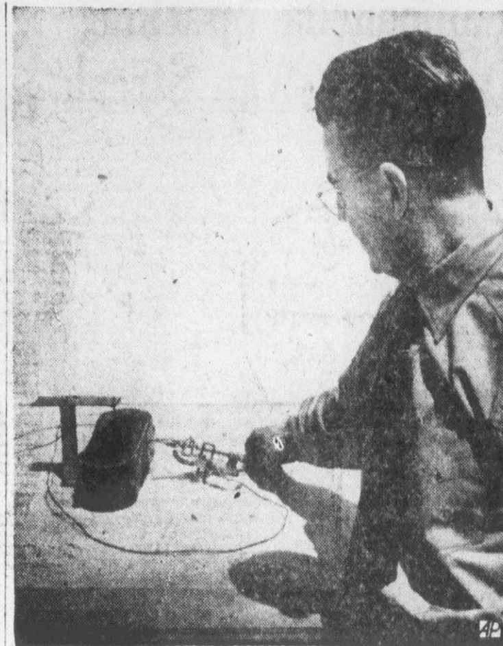
SOLAR GENERATOR—Lt. Col. Gerard M. Leies, one of the two men who discovered cadmium sulfide, best transducer known to date, adjusts the position of a solar generator to enable it to catch the maximum amount of light. The machine, developed at the Air Research and Development Command's Wright Air Development Center at Dayton, O., produces 1-3 of a volt in this model. When refined, the Air Force said, the machine could light an entire home. (Air Force Photo via AP Wirephoto)
