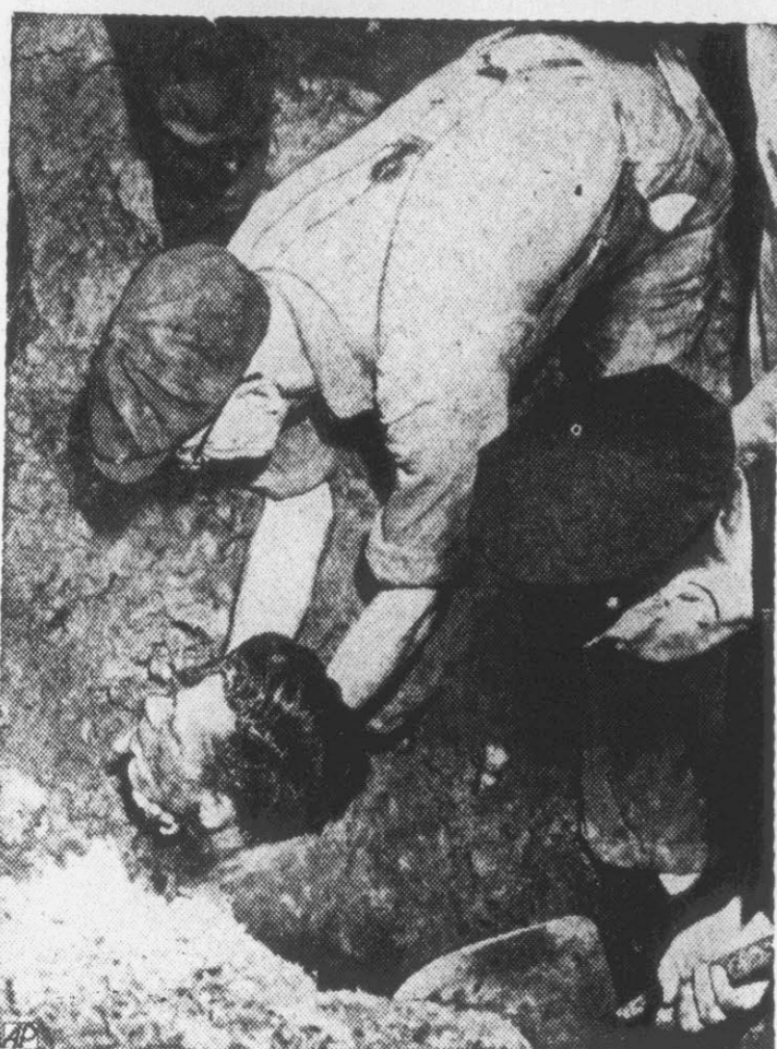
Rescuers dig soft mud from around Stanley W. Pakel Jr. of Johnson City, N. Y. after he was trapped and completely covered by a cave-in in the ditch in which he was preparing to lay a sewer pipe in Binghamton, N. Y. Fellow workers used their hands to dig the mud from around his head to keep him from suffocating. (AP Wirephoto)
