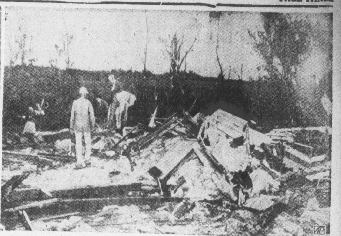
TORNADOES BRING RUIN—Neighbors and members of the Gene DeRoot family probe the ruins of the DeRoot farm home at Norfolk, Nebraska, after a tornado ruined several homes in the area. Several tornadoes cut a swath across the northeast part of the state killing four children and injuring at least 18 other persons. (AP Wirephoto)
