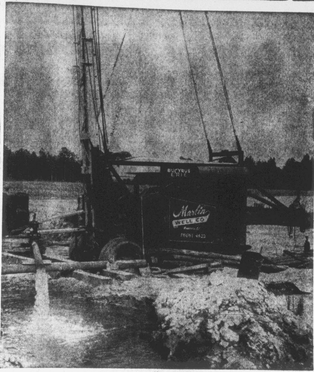
The above picture shows water flowing from the recently dug well on the Langston farm. A total of 120,000 gallons were pumped from the well in eight hours for an average of 250 gallons per minute. It is estimated that that amount of water is enough to put more than an inch on four acres of tobacco. (Reflector photos by Alvin Taylor)
