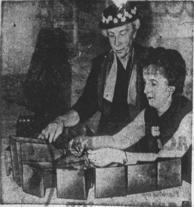
TIME-SAVER. Dr. Lillian Gilbreth, left, shows Anna Stanchek, Newark College of Engineering student, how bins save time and effort in assembling antennae.
