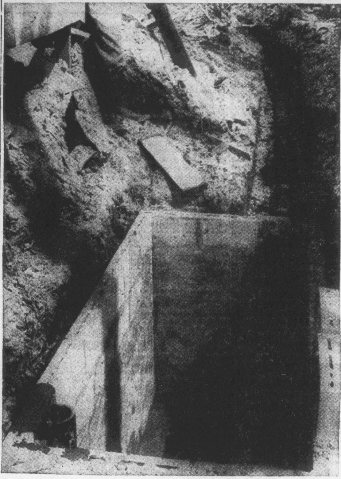
Here is a homemade concrete block septic tank located on a Pitt County farm. With this type tank a farm can be equipped with all the city conveniences in the country. This is the type of tank recommended by the Pitt Health Department. Information and help on construction of this type tank can be obtained from the Health Department. (Reflector Staff Photos by Bob Boyette)
