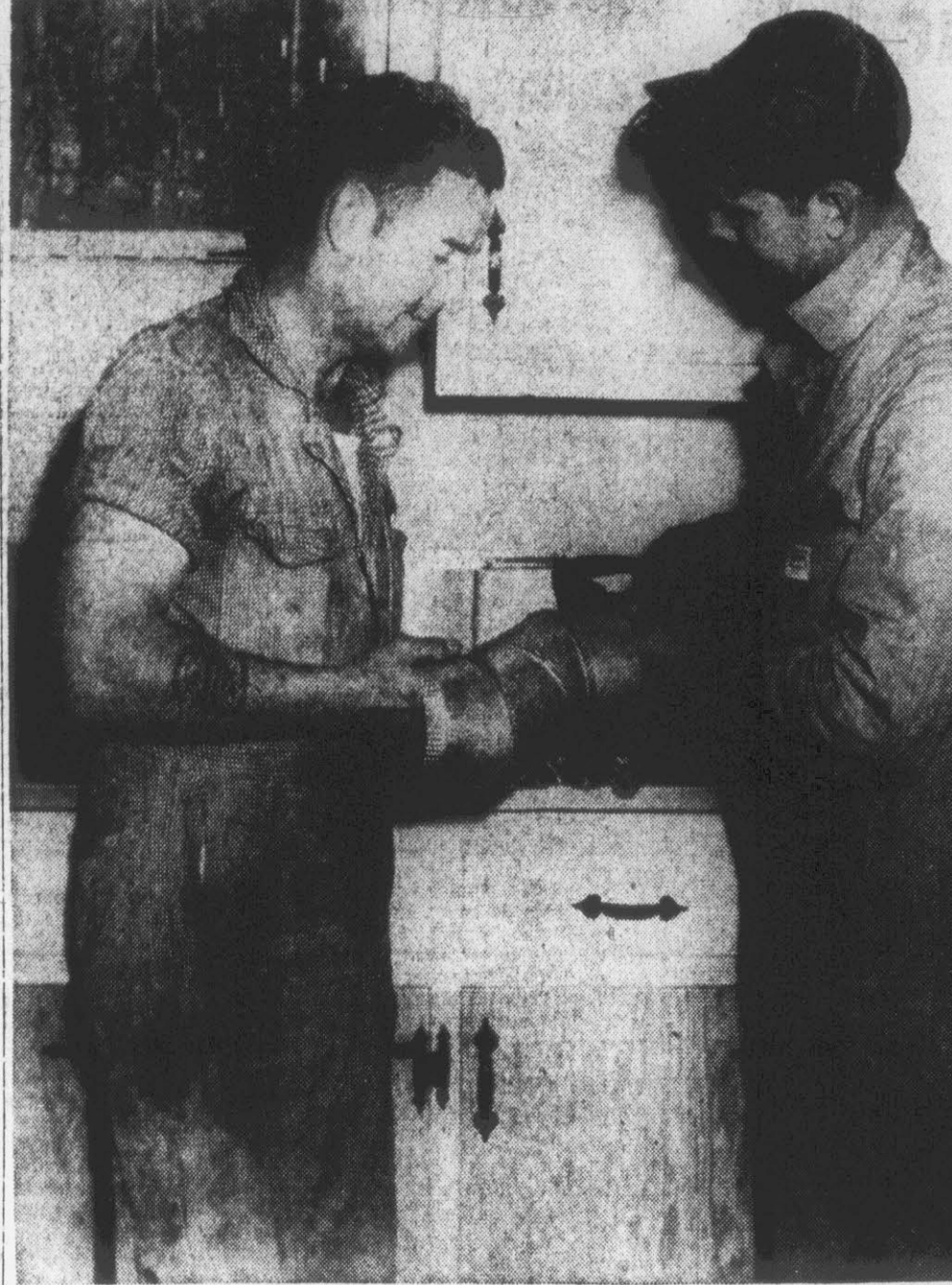
Shown above are two workmen as they put the finishing touches on a kitchen in the new recreation building at Elm Street Park. The workmen installed sinks and other equipment in the kitchen. The recreation building is being completed with labor and materials which is being donated by local business firms. (Reflector photo by Alvin Taylor)
