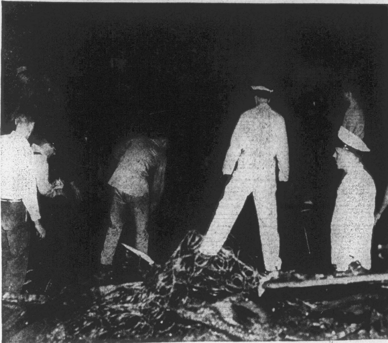
Pictured above are rescue workers as they probe the wreckage of a furniture store which was completely destroyed by a terrific explosion in Goldsboro yesterday. Workmen dug out the third of five bodies which have been found so far just after this picture was taken at 7:00 o'clock last night. The rescue operations went on far into the night with volunteers working by floodlights. Out-of-town fire-fighting units assisted the Goldsboro Fire Department. (Photo by C. L. Perkins Jr.)
