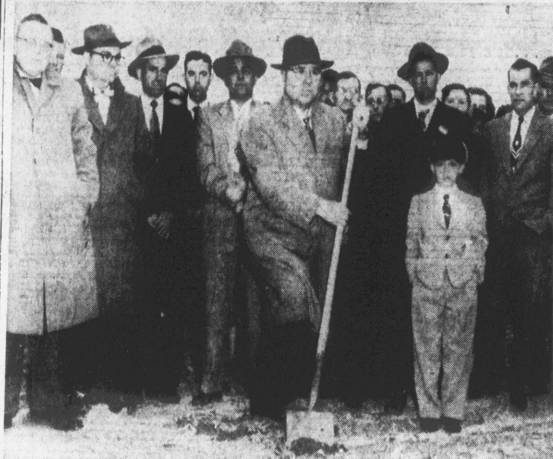
GROUND BREAKING CEREMONIES—Rev. Rashie Kennedy (center), pastor of the new Grace Free Will Baptist Church in Greenville, broke ground for the new church building in ceremonies here Sunday afternoon. The ceremonies were held at the site of the new church at the corner of Watauga Ave. and Spruce Street. Construction on the new building began yesterday. The first unit of the new church to be constructed will consist of a 40 by 100 foot structure which will be used for both Sunday School and worship services. Plans call for the addition of a sanctuary later. At the extreme left in the picture above is the Rev. Hubert Burress of Saratoga, secretary-treasurer of the Central Conference Mission Board of the Free Will Baptist Church, who attended the ceremonies. (Photo by Roy Hardee)
