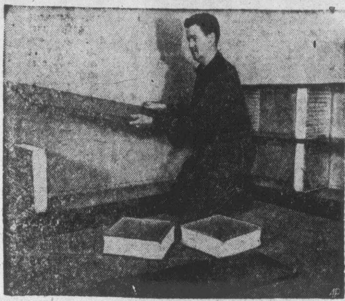
AP Newsfeatures ATTRACTIVE CORNER book shelves are easy to build merely by stacking boards on glass blocks. Two or three coats of paint will give the shelves a suitable finish.
