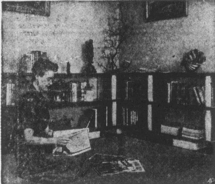
THE FINISHED SHELVES add a smart modern note to the room. You need have no worry about the strength of the shelves, because the glass blocks used are made for structural use. Blocks laid on their sides raise the bottom shelf from the floor. The shelves are easily dismantled and moved.
