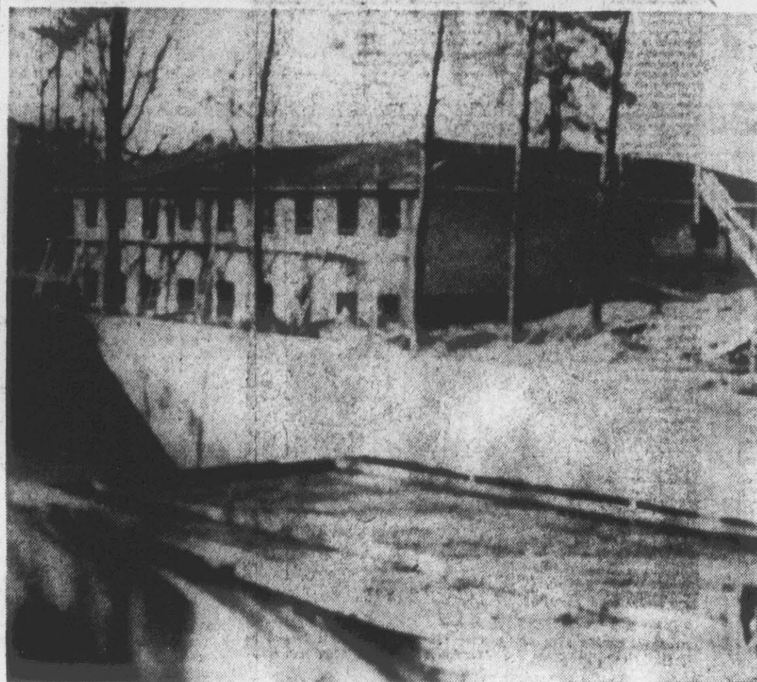
Pictured above is a view of the new swimming pool and locker house which are now being constructed at the Greenville Country Club. The pool itself is being built at a cost of $19,000 and measures 30 feet by 75 feet. It will be nine and one-half feet deep at its deepest point. In addition, a 20 by 20 foot wading pool is being constructed by the Country Club. Cost of the locker rooms will be approximately $15,000 and space will be provided for 200 lockers. Dr. Dan Wright, president of the club, said that it is planned to open the pool sometime in May. (Reflector photo by Alvin Taylor)
