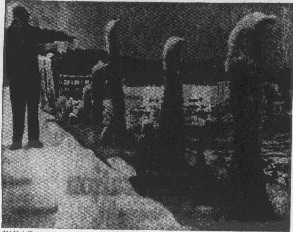
WHAT ARE THEY? — Air pipes put beneath water to prevent ice damage to shaft board of Gulf Island Dam, Lewiston, Me., cause ice to build up on surface in these formations.
