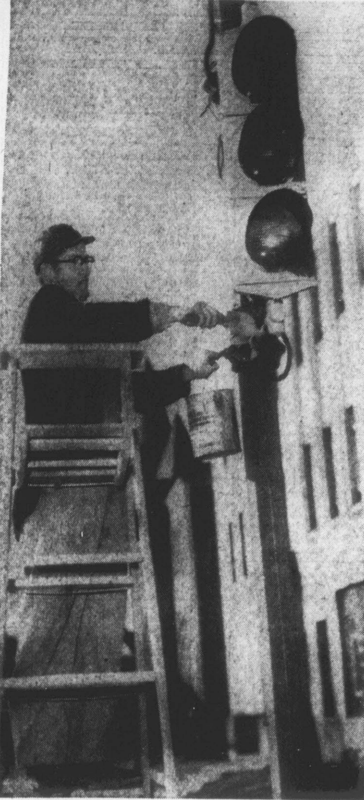
Street department workers were busy this morning giving the city's stoplights a new coat of yellow paint. City Manager James S. Hughes said that yellow will be used principally for visibility and that all the traffic lights in Greenville will be painted that color. Hughes noted that yellow is getting to be the standard color for stoplights all over the country. The above picture was taken at the corner of Fifth and Washington Streets. (Reflector photo by Alvin Taylor)
