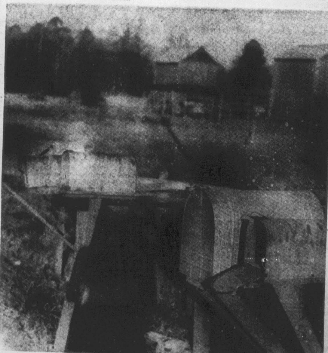
One of the rural mail carrier's pet peeves are mail boxes which are not installed according to postal regulations. Some of the above boxes are sagging and others are propped up. On many boxes the door latches will not fasten.
