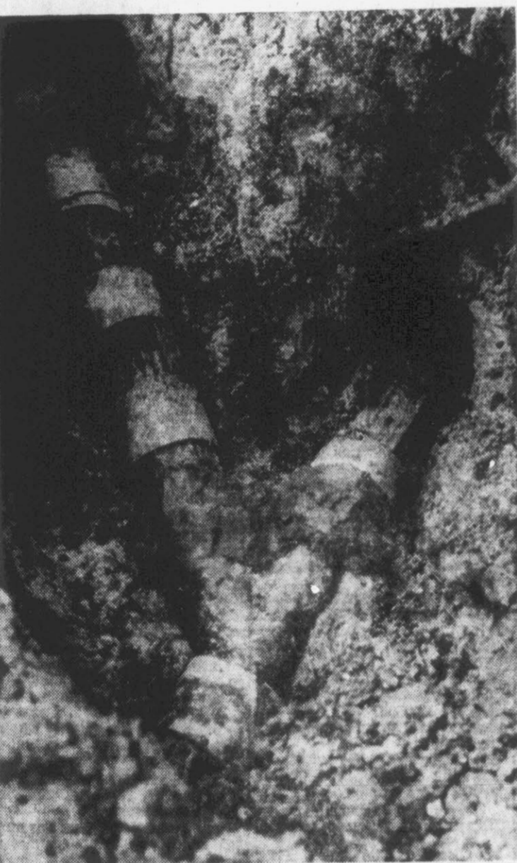
Above is a "Y" joint used to connect two lines of tile. In this way an entire field can be connected to drain into a ditch or stream. Each joint of the tile line is covered with a strip of tar paper to prevent dirt from seeping into the line.
