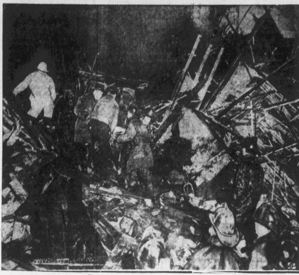
TRAPPED BY COLLAPSE:—Firemen remove a fellow fire fighter from the ruins of a building at 1702 West Madison Street in Chicago after he and several others were trapped when the entire front of the building collapsed following a pre-dawn fire. Tenants fled from the blaze of the 3-story West Side hotel into near zero cold. (AP Wirephoto).
