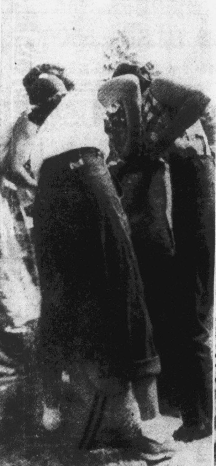
Ladies of Grifton spread 600 pounds of salt on the tennis court area at the new park. The salt is to prevent weeds and grass from growing up on the tennis courts after they are paved.
