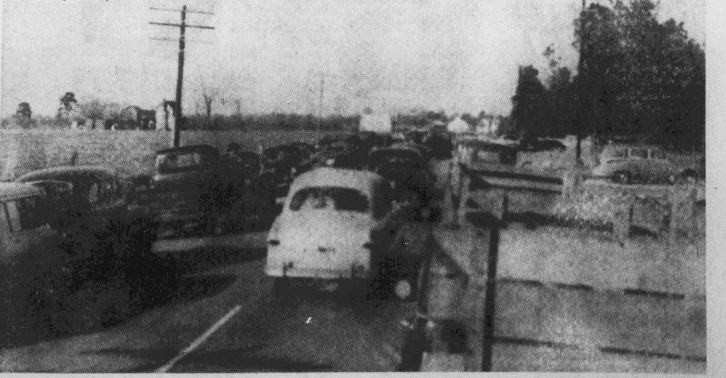
A virtual traffic jam was created yesterday on Evans Street Extension in front of television station WNCT when large numbers of motorists stopped to watch tower construction from the road. Highway patrolmen had just begun to order drivers to move on when this picture was taken. Later in the day "No Parking" signs were installed along the road by the highway department. (Reflector Photo by Alvin Taylor)
