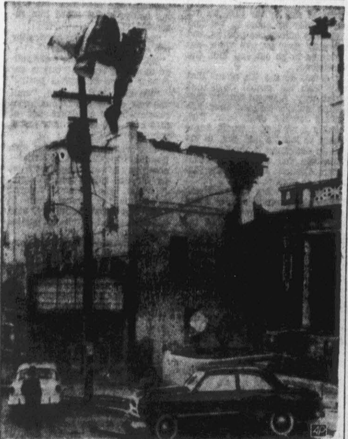
TORNADO TRAPPED 73 —A vicious tornado struck Vicksburg, Miss., and collapsed the roof of the Saenger Theatre and trapped 73 persons, 34 of whom were children. Rescue gangs were working in freezing weather in a grisly hunt for additional victims of the blow that took at least 30 lives. National Guardsmen on guard duty built fires from the debris that littered the streets. (AP Wirephoto).
