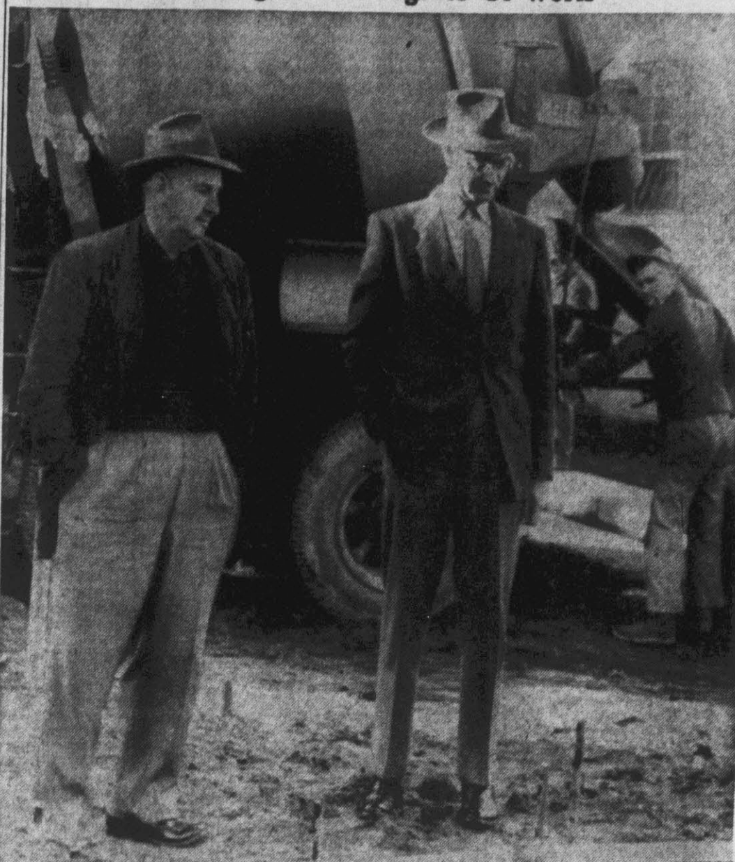
Street Superintendent O. K. Beatty, left, and City Manager James S. Hughes inspect the new curb being laid today to enlarge the parking area between the Municipal Building and the Fire Station. The additional space will allow ten more cars to park there. A total of 21 parking spaces will be in that area when this work is completed. Hughes said he hoped that the area would be graded by early next week. The City Council approved the enlarging at their last meeting. (Reflector Staff Photo by Bob Boyette).
