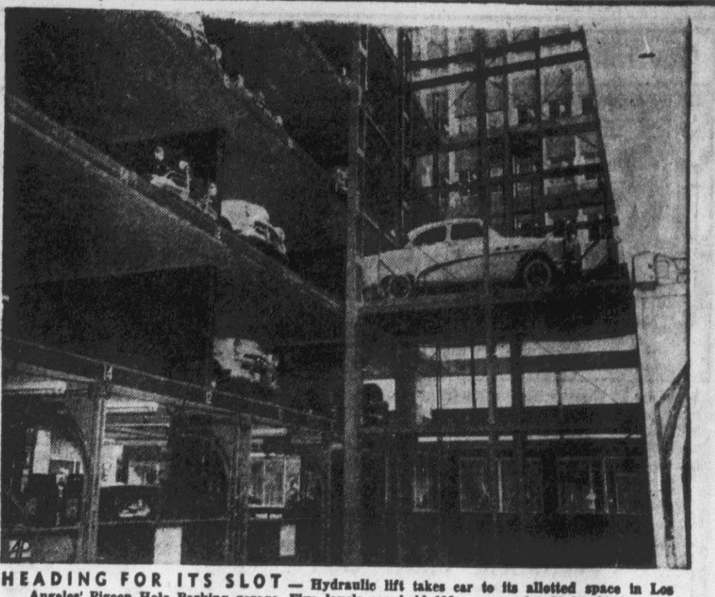
HEADING FOR ITS SLOT — Hydraulic lift takes car to its allotted space in Los Angeles' Pigeon Hole Parking garage. Five levels can hold 128 cars on plot 60 by 90 feet.
