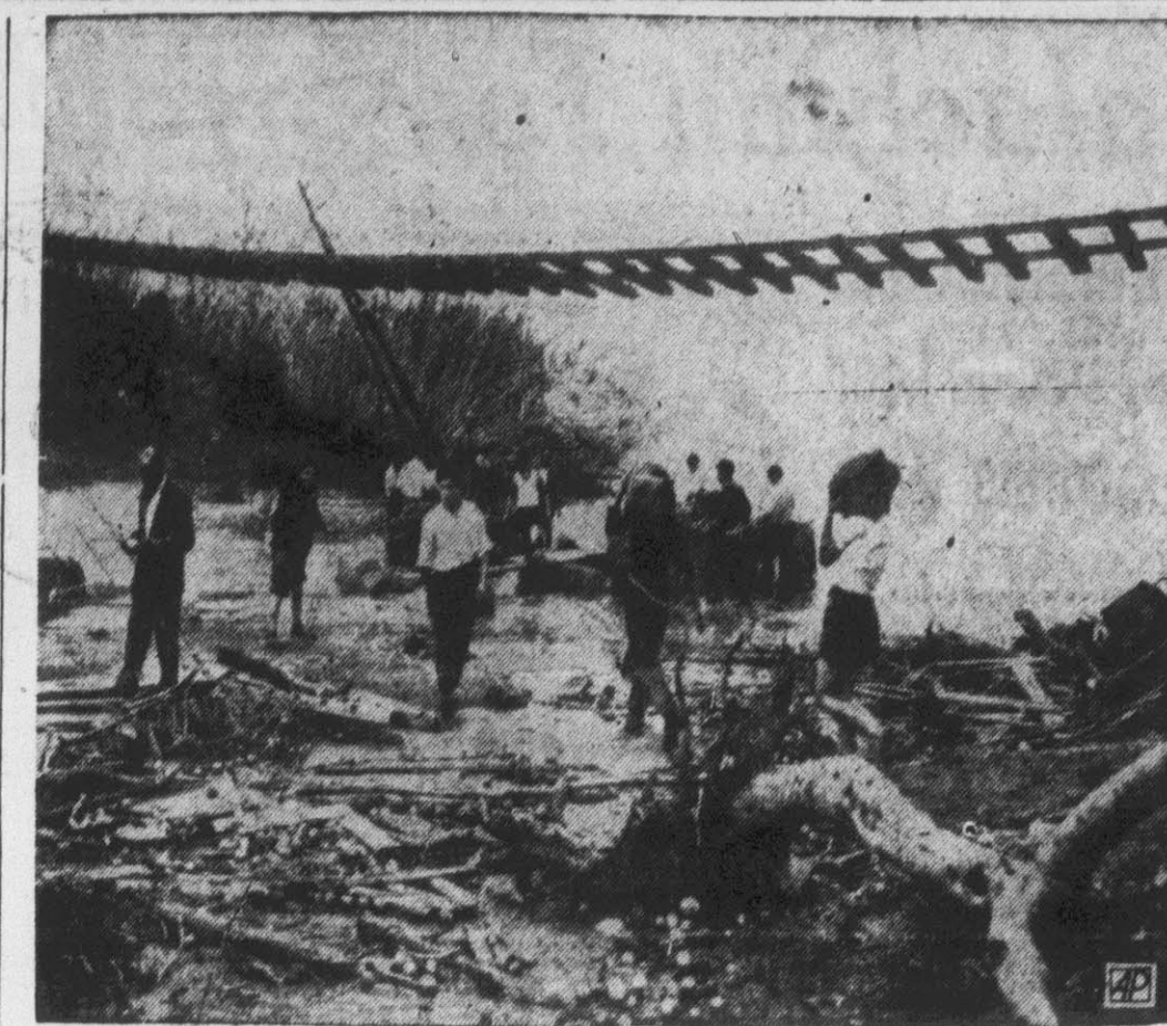
FLOODS WASH AWAY BRIDGE—A railway track sags after bridge on which it ran was swept away in severe floods in the Calabria region of southern Italy. The bridge stood at San Gregorio, a small town near Reggio. Heavy rains are falling throughout the province where floods in the past week caused 58 known deaths and wrought heavy damage. Volunteers attempt to clear away debris. (AP Wirephoto).
