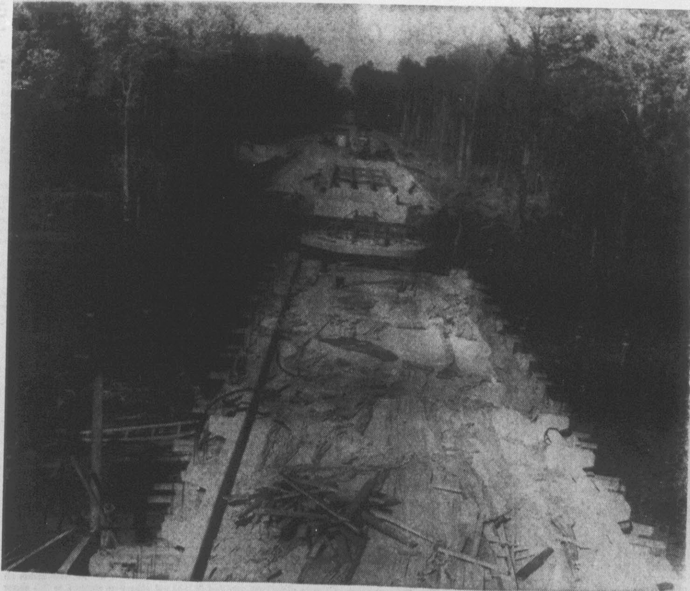
Construction on the new Grimesland River bridge, which will span the Tar just below Grimesland, is moving along at a good pace. Work on the bridge was begun months ago and is scheduled to take around a year to complete, along with the construction of a new road leading to the site.
