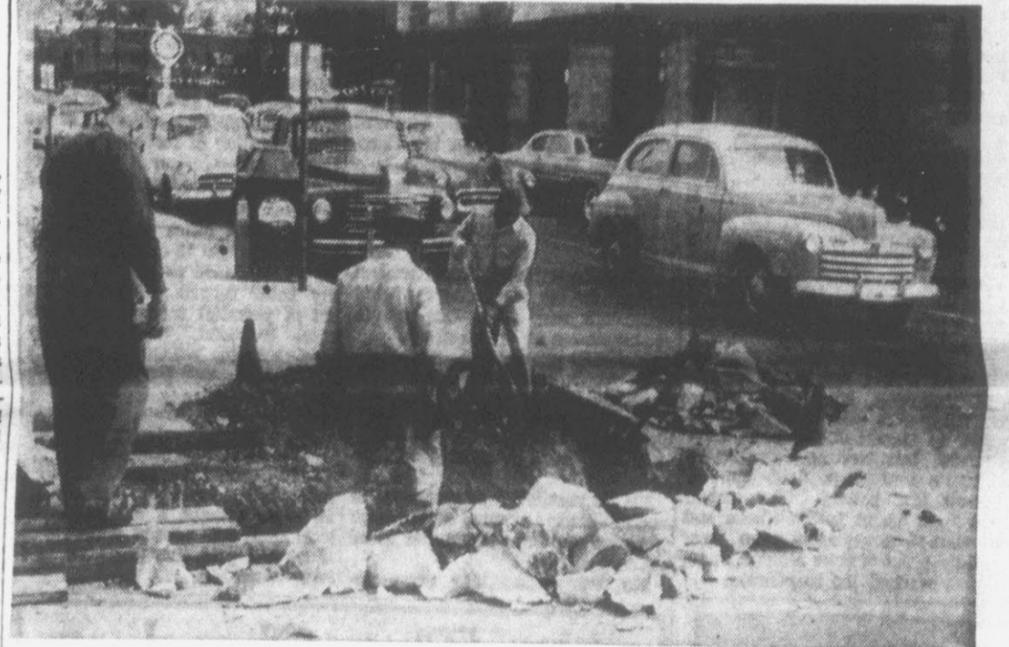
STREET REPAIR WORK—Street Superintendent C. K. Besty is shown supervising the work of one of his crews which have been engaged in the reworking of streets and sidewalks in Greenville. Several sections of uptown sidewalk, crumbled and "ragged" for years, have been removed and replaced with newly-poured cement. (Reflector Photo by Roy Hardee)
