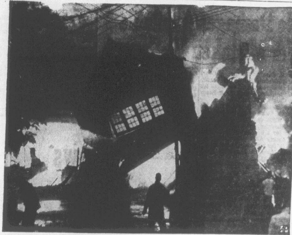
WAREHOUSE WALL TOPPLES.—Wall of Lexington, Ky., tobacco warehouse falls amid flames that caused $350,000 loss to warehouse and 20 nearby buildings and homes.
