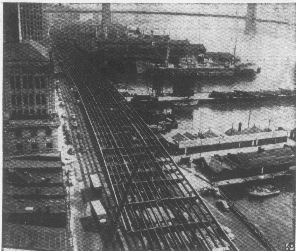
HIGHWAY SKELETON — Steel frame for stretch of elevated highway along New York's East River is completed. It will link with roads circling Manhattan's 24 mile perimeter.
