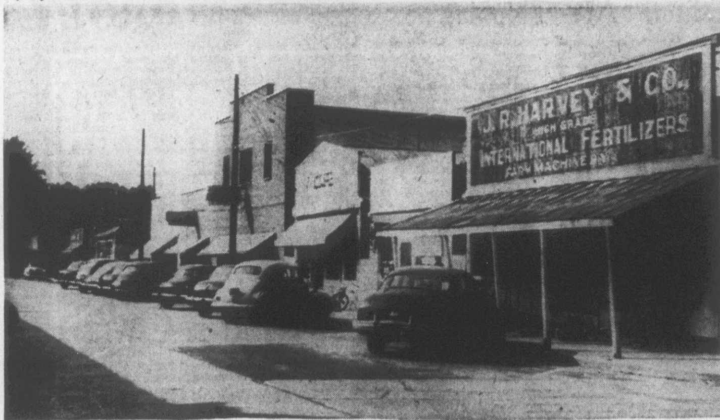
Here is a downtown view of ever growing Grifton. Before the construction of the large DuPont plant near Grifton began, the town had made very little progress in keeping up with the rest of the Eastern part of the state. However, in a matter of weeks it was turned into a regular boom town with new stores constructed and housing projects.
