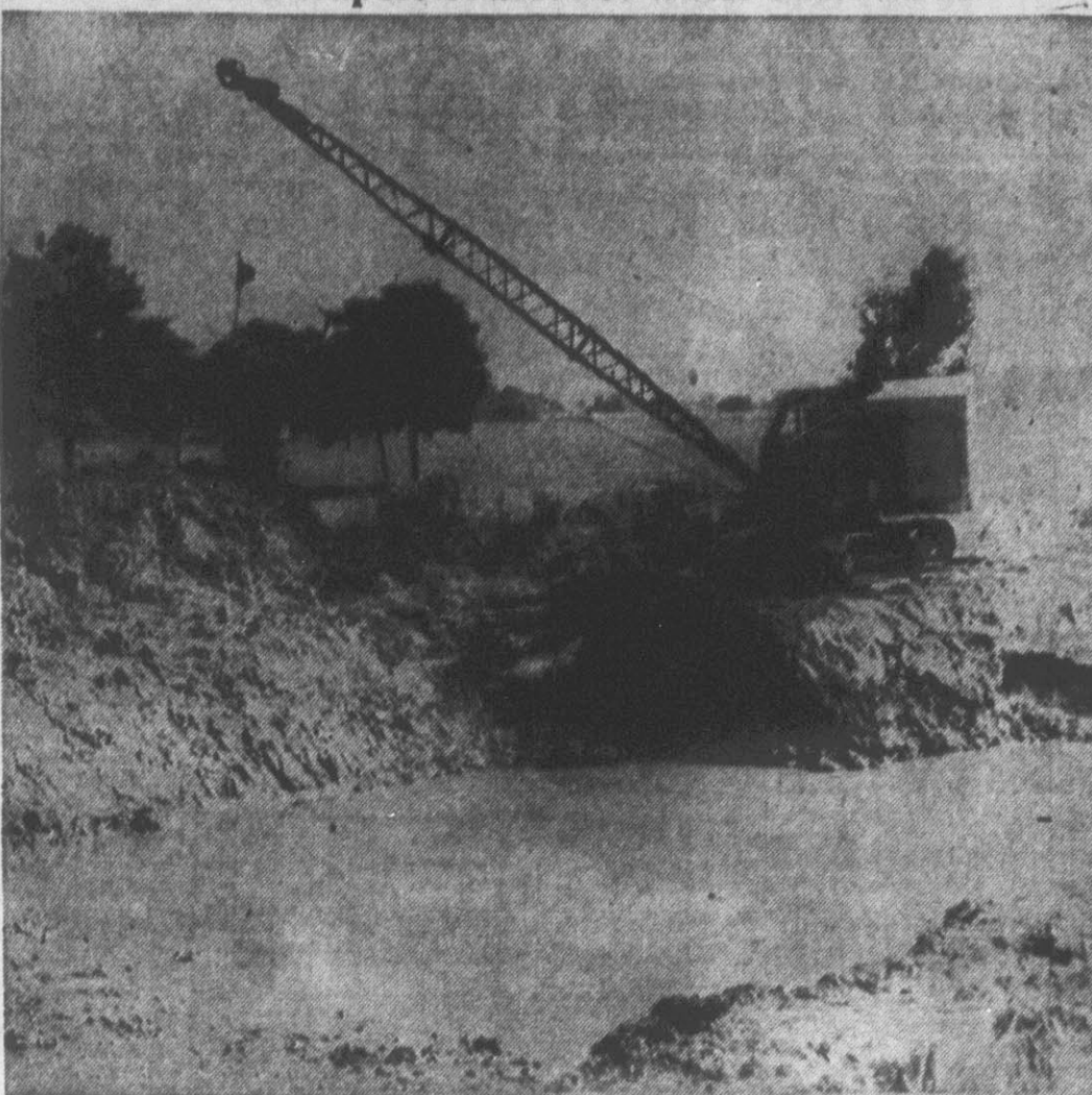
This water hole in W. R. Eagles 100-acre pasture in the Tar River second bottom above Falkland furnishes an ample supply of water for his 75 cattle. Water is one of the most important and cheapest requirements for livestock, and with this 12-foot deep, sloped water hole the cows in Eagles' pasture will never be without the necessity. The hole is 60 feet wide and 100 feet long and is sloped so that the cattle can walk to the edge no matter how low the supply of water is. Twelve of these holes have been dug by the Hoke dragnine in the past 30 days. (Reflector photo by Tommie Lupton).
