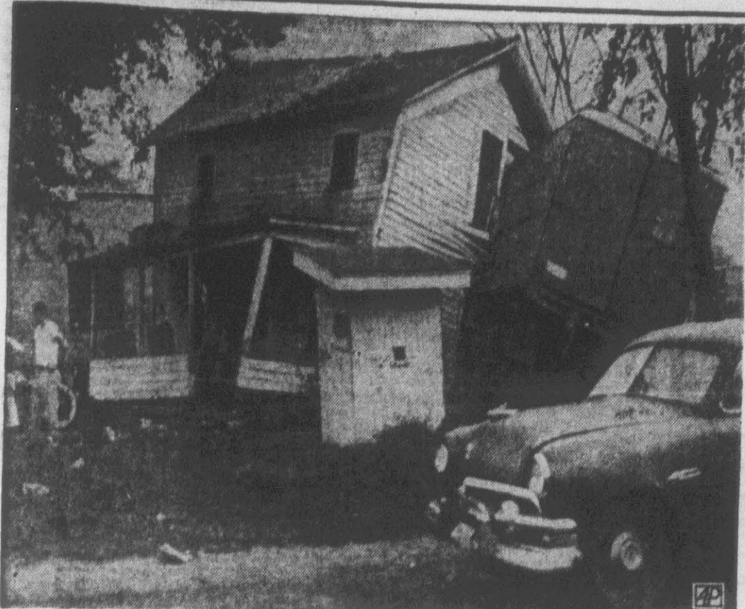
TRUCK CRASHES HOUSE—A man and his wife were killed while asleep in a first floor bedroom of this house at Havana, Ill., when a big trailer-truck crashed into the structure virtually demolishing it. Dead by Attorney John Hurley said the truck driver, Don Kelling, apparently dozed at the wheel. He was not held. AP Wirephoto
