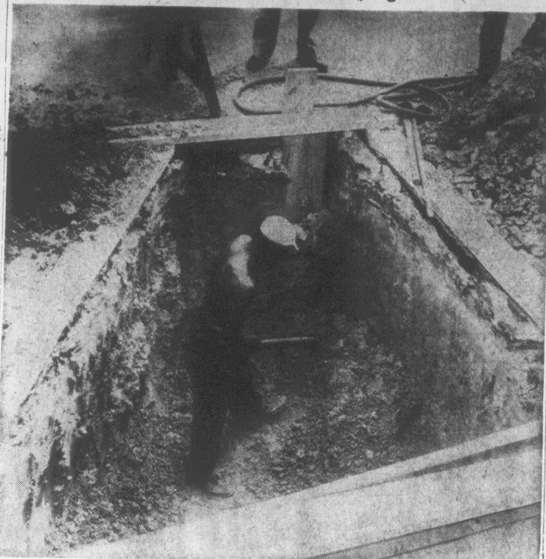
Construction workers have begun to make progress in preparing for the laying of the cable which will carry network television programs to Greenville Television station when it goes into operation. The work above was being carried on at Fifth and Pitt Street where the cable will start and then go out to Evans Street to the site of the TV station. (Reflector Photo by Roy Hardee)
