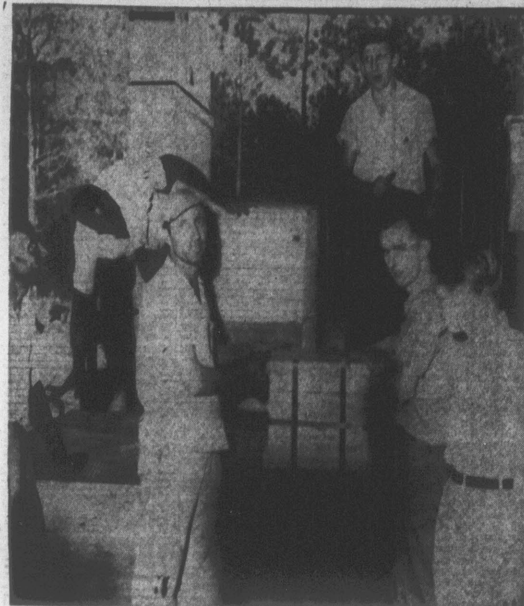
Workers are shown above as they were unloading the transmitting equipment yesterday afternoon at the Greenville Television Station. Earlier in the week crews of the Carolina Telephone and Telegraph Company began construction work on the cable to bring network television programs here. (Photo by C. L. Perkins, Jr.)
