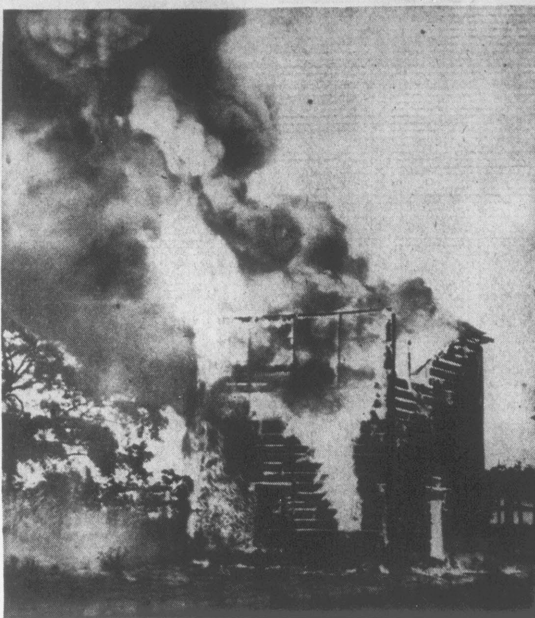
Angry flames and smoke shoot skyward from the blazing tobacco barn shown above as the product of many months of hard toil goes up in ashes. The tobacco barn and its contents pictured above belonging to Edmond Speight and located on the Elmer Holmes farm near Kings Cross Road was destroyed by fire Saturday afternoon. The picture above was made soon after the fire started by Patrolman D. E. Perry of Bethel.
