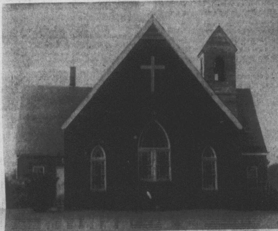
AT BALLARDS CROSSROADS—After first holding services in a school building, Presbyterians at Ballard's Crossroads on Highway 264 southwest of Greenville constructed the handsome brick sanctuary and educational building above. Organized in 1944, the church now has 96 on its rolls. A Sunday School in this community was held as early as 1905.
