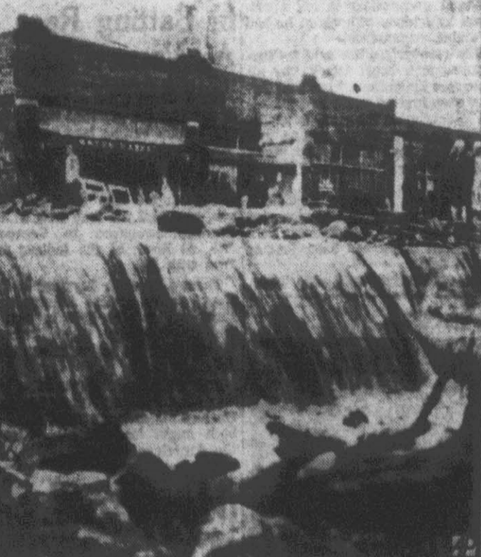
MAIN STREET.—Floodwaters pour over a six-foot ledge gouged in Bayfield, Wisconsin's main street as a result of heavy rain. The torrent caused an earthen dam at the reservoir on the edge of town to give way, sending an avalanche of water into town. No one was injured, but damage was estimated at $100,000. (AP Wirephoto)
