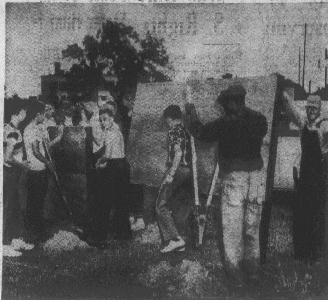
Boys in the Pony League are shown as they help construct a fence around a field at Third Street School. The field will be used by the City Softball League on Monday, Wednesday and Friday nights and the Pony League on Tuesday and Thursday nights. Lights are supposed to be up by Monday and play in the league is scheduled to begin at that time.
